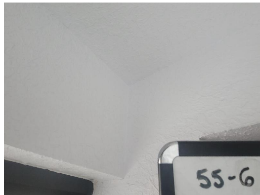
55-6 Drywall/Joint Compound Typical Interior Walls/Ceilings
