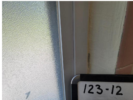
123-12 Caulk Typical Interior Windows
