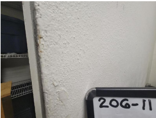
206-11 Plaster Typical Interior Walls/Ceilings
