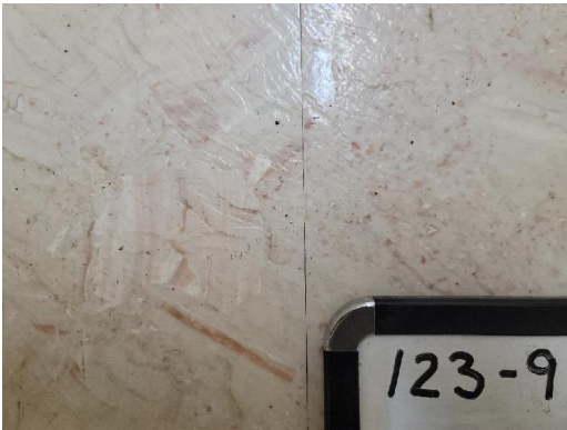
123-9 12"x12" Floor Tile/Adhesive Interior Bathroom Edges
