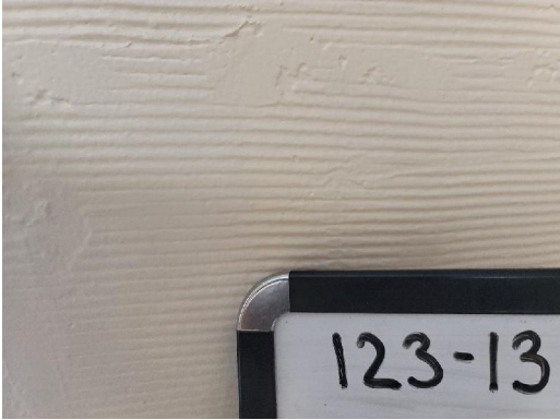
123-13 Wall Tile Mastic Interior Kitchen
