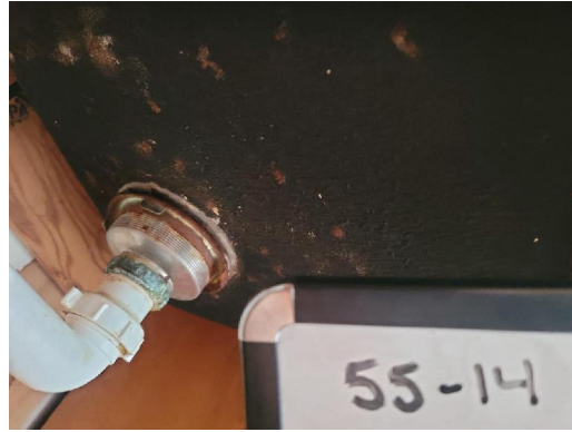
55-14 Sink Mastic/Black Interior Kitchen 4% Chrysotile
