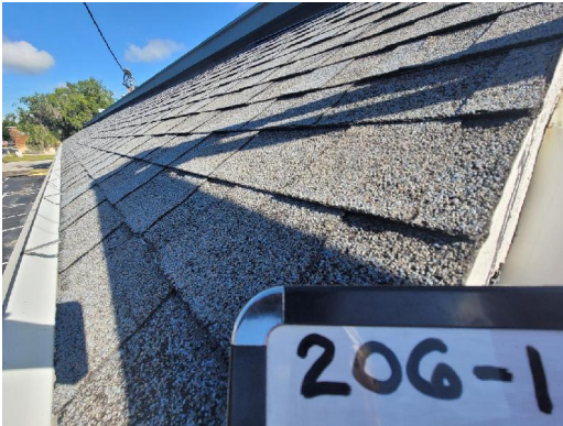
206-1 Asphalt Shingle/Tar Exterior Roof Overhangs
