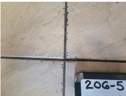
206-5 Grout Interior Rear Entry Tile Flooring
