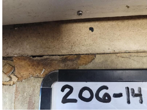
206-14 Rolled Vinyl Flooring/Brown Typical Interior Main/Bottom Layer 17% Chrysotile/Appx 1,320 sq. ft.
