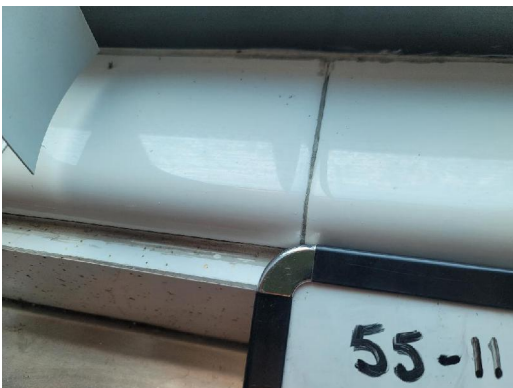
55-11 Grout Typical Interior Window Sill Tile
