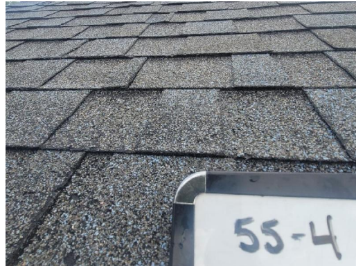
55-4 Asphalt Shingle/Tar Typical Exterior Peaked Roof
