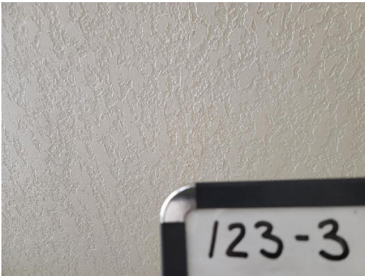
123-3 Drywall/Joint Compound Typical Interior Ceilings
