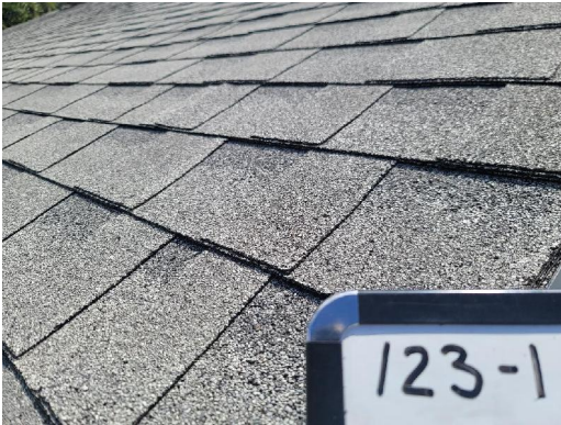
123-1 Asphalt Shingle/Tar Typical Exterior Roof
