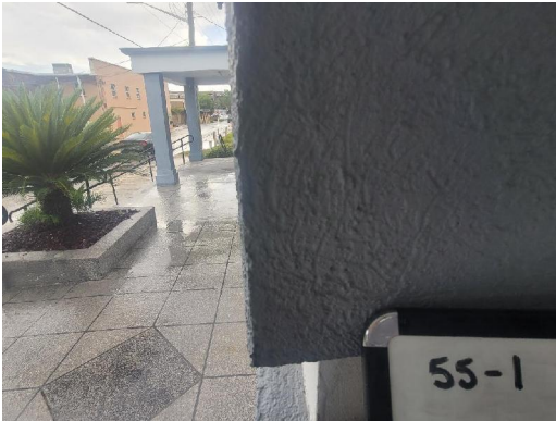
55-1 Stucco Typical Exterior Walls/Windows
