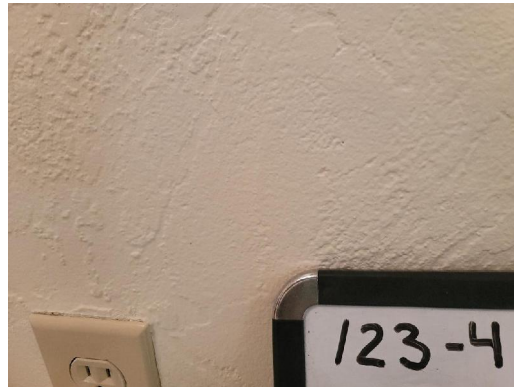
123-4 Plaster Typical Interior Walls
