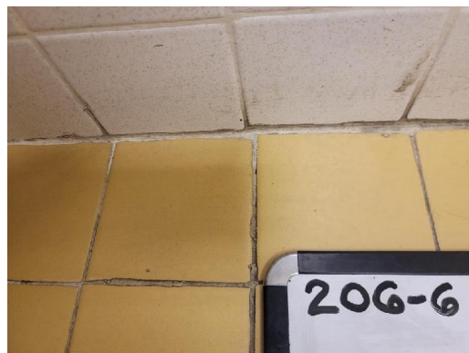
206-6 Grout Typical Interior Men's/Women's Rooms Wall/Floor Tile
