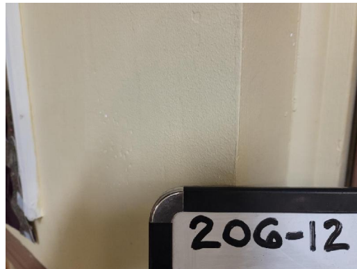
206-12 Drywall/Joint Compound Typical Interior Walls
