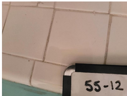
55-12 Grout Interior Baptismal Pool Tile
