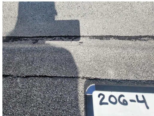
206-4 Rolled Asphalt Roofing/Tar Typical Exterior Main Roof
