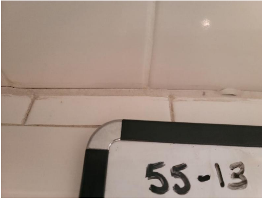
55-13 Caulk Interior Baptismal Pool Tile
