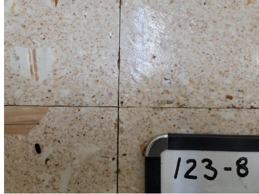
123-8 12"x12" Floor Tile/Adhesive Interior Bathroom
