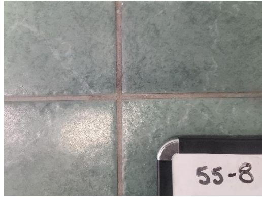
55-8 Grout Typical Interior Hall Tile Flooring
