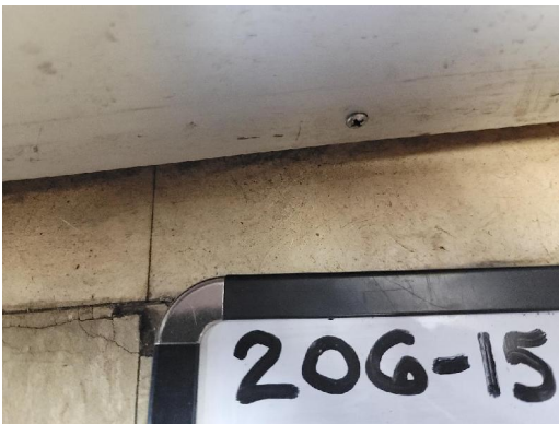
206-15 12"x12" Floor Tile/Adhesive Interior Office
