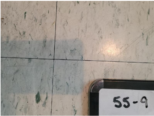
55-9 12"x12" Floor Tile/Mastic Interior Chapel/Kitchen
