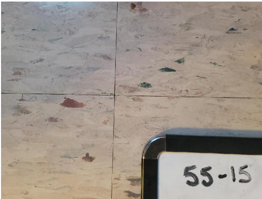
55-15 12"x12" Floor Tile/Mastic Interior North Women's Room
