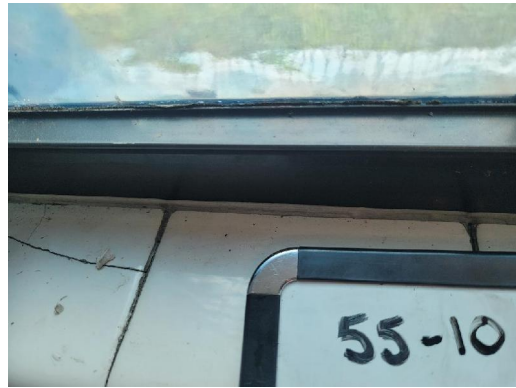
55-10 Caulk Typical Interior Windows
