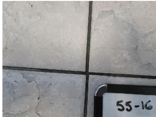
55-16 Grout Interior North Men's Room Tile Flooring
